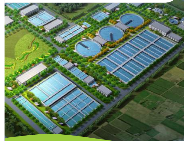
泰兴经济开发区污水处理厂 Taixing Economic Development Zone WWTP
