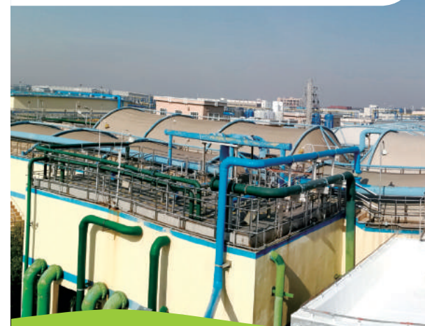
上海化工园区污水处理项目 Shanghai chemical industry park wastewater treatment project
